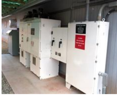
Figure 5. String inverter. Photo by Warren Gretz, NREL 07985
