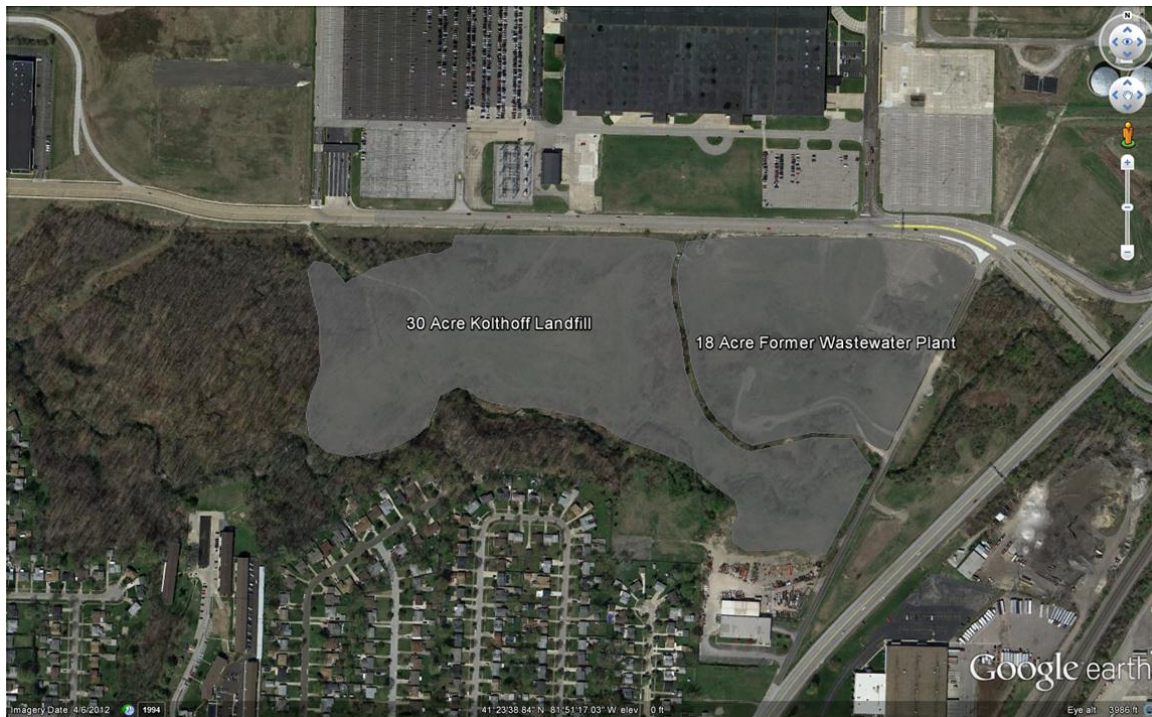
Figure 6. Aerial view of the Kolthoff Landfill and former wastewater plant (shaded in gray)
