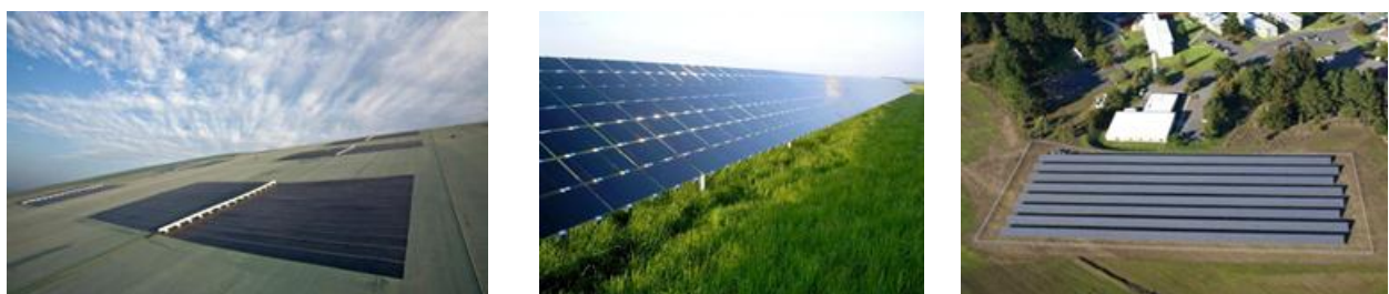
Figure 4. Thin-film solar panels installed on (left) solar energy cover and (middle/right) fixed-tilt mounting system. Pictures from (left) Republic Services, Inc., NREL 23817; (middle) Beck Energy, NREL 14726; and (right) U.S. Coast Guard Petaluma site, NREL 17395
